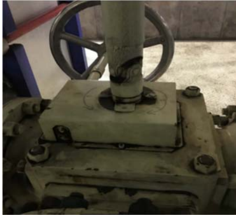
Figure 13. Sharpie inscribed 6-way transfer valve position indication as found. 43
